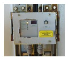
In addition, Fire Suppression Gas Release Status Units made of pressed mild steel, exposed to the sea conditions have been seen to deteriorate. Even when these units are made of stainless steel they continue to use ABS plastic components which perish with the harsh conditions.
